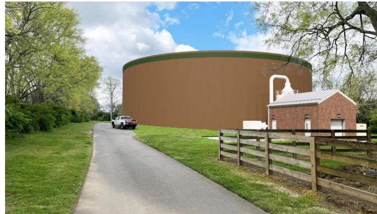
Partially Buried Option – Sidewall 35 ft above grade on Concord Road side
