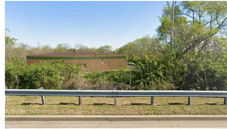
Partially Buried Option – Sidewall 15 ft above grade on Concord Road side
