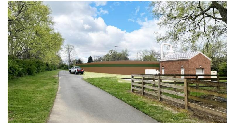
Deeper Bury Option – Sidewall 3 ft above grade on Concord Road side
