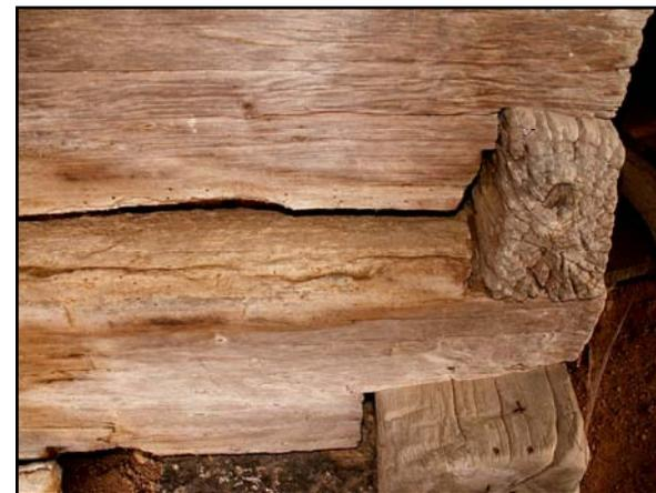
*Log barn construction using half-dovetail design was of Germanic origin*
